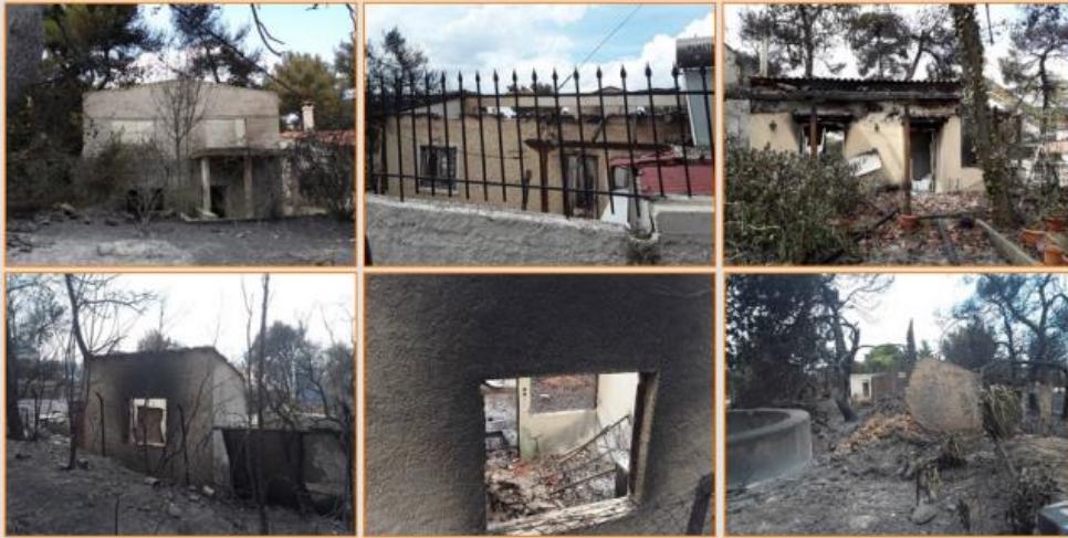
Various damage on masonry buildings with load-bearing masonry walls ranging from destruction of external and internal combustible contents induced by firebrands attack, radiant heat exposure and/or flame contact, to partial collapse of the building
